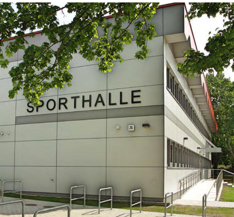
© Boening | Sporthalle Hagenstraße
