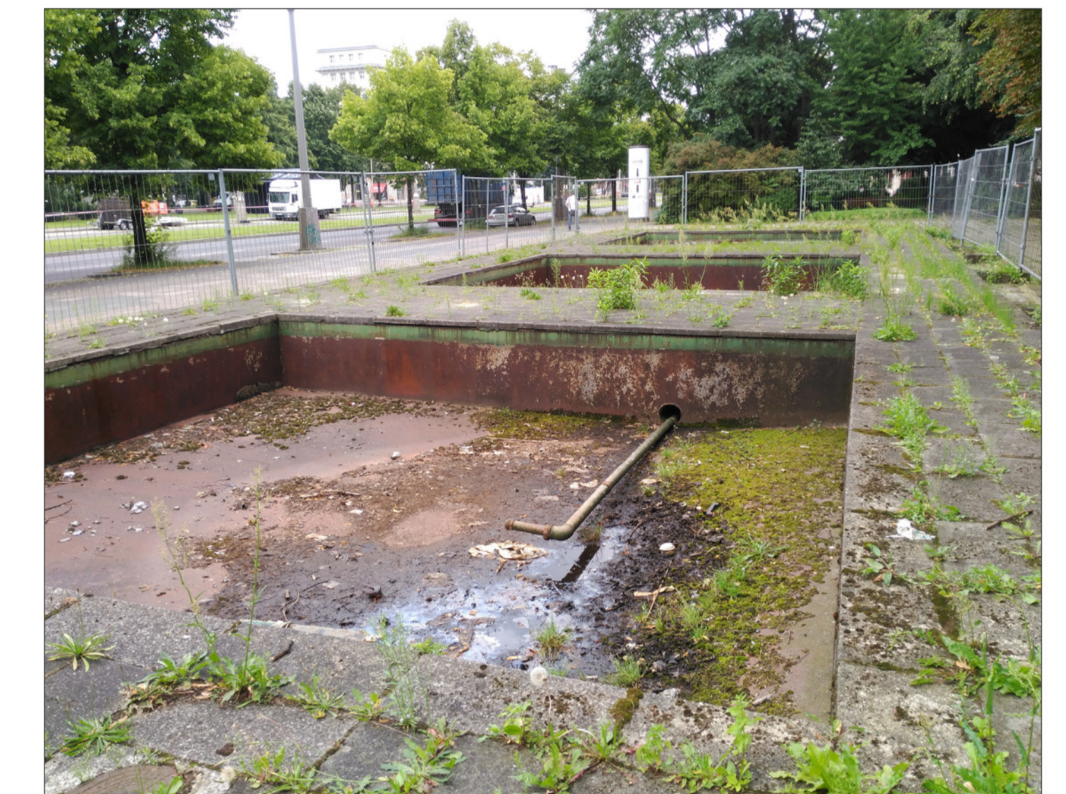
Blick in Richtung Westen - August 2017
